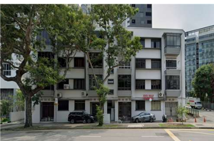
River Valley Apartments
