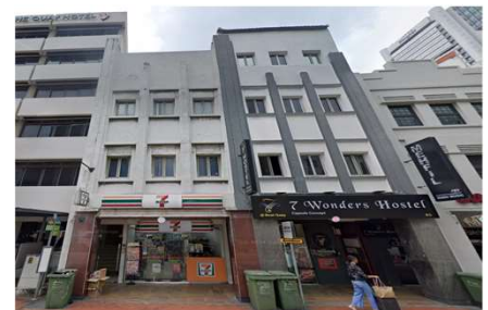
63 & 65 South Bridge Road
